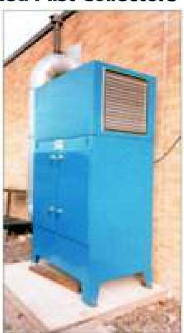
cabinet where it may be easily removed through the 3/4" BSP drain hole. If desired, collected coolants can be recycled by connecting the mist filter drain to the machine coolant system with a 'U' trap arrangement. 3rd stage absolute filter is only required where smoke penetrates the high-efficiency 2nd stage fibreglass filter.
